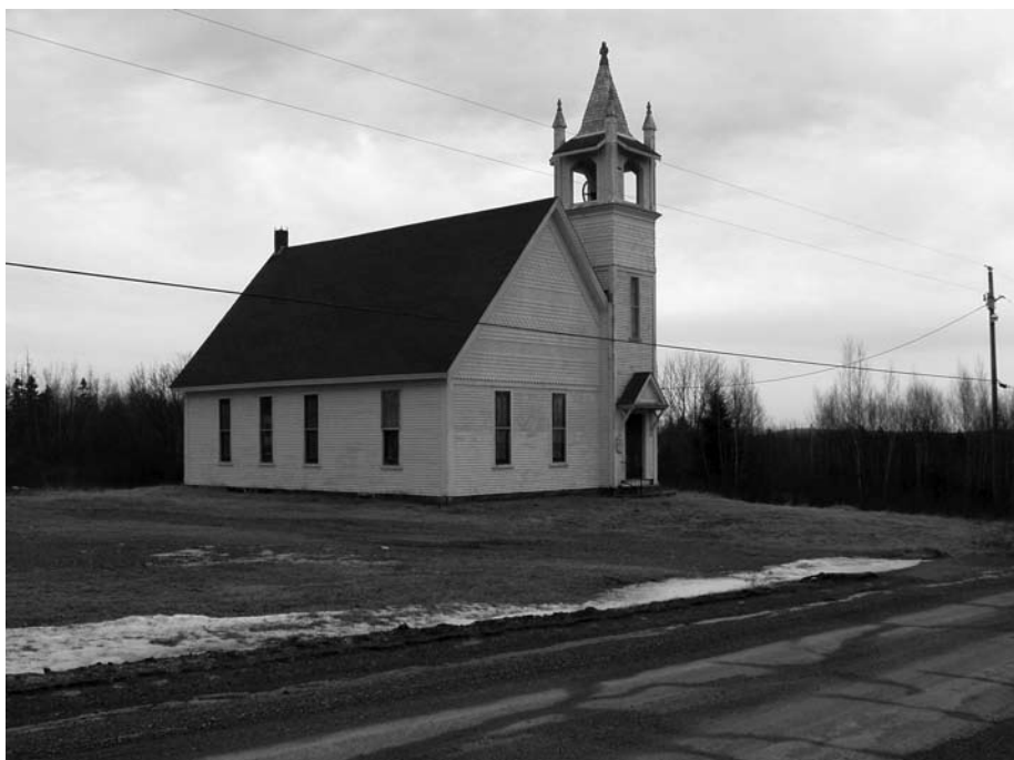
The Congregational Church closed about ten years ago, and the building is no longer in use.
