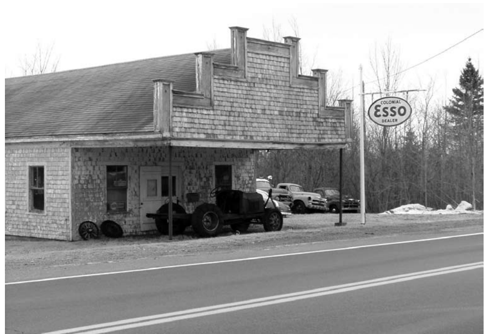
This old service station, built by Lloyd S. Williams, was originally a repair garage and filling station. Built in 1935 on the site of David DeLong's store, which burned in 1932, Lloyd operated his service station until 1942. He opened it again from 1945-1952, and again from 1956-1963, before turning it into an antique shop in 1976.
